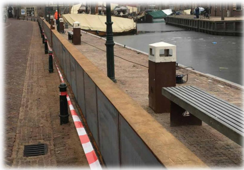
Figure 60: Automatic sea wall technology (Image Source: The Flood Company, Flood Control International)
