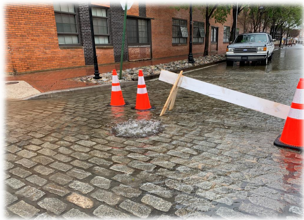
Figure 26: Nuisance flooding and stormwater system backflow along Thames Street In May 2020. The northwest branch Patapsco River tidal gauge registered a 4.3 feet tide high during this period
